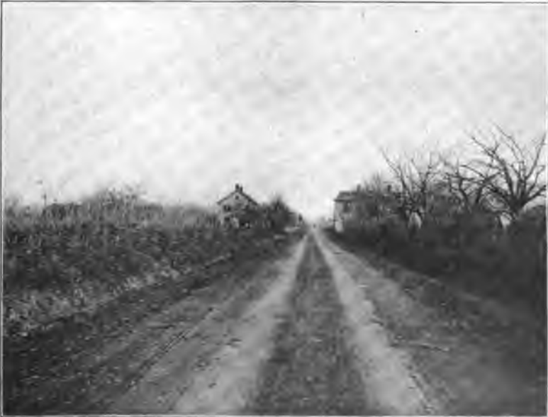
Neshanic road, Somerset Co., after improvement.
